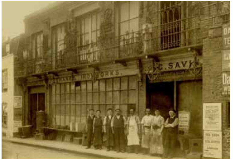
Stevens ironworks at No. 36 King Street (1890) © Margate Civic Society
