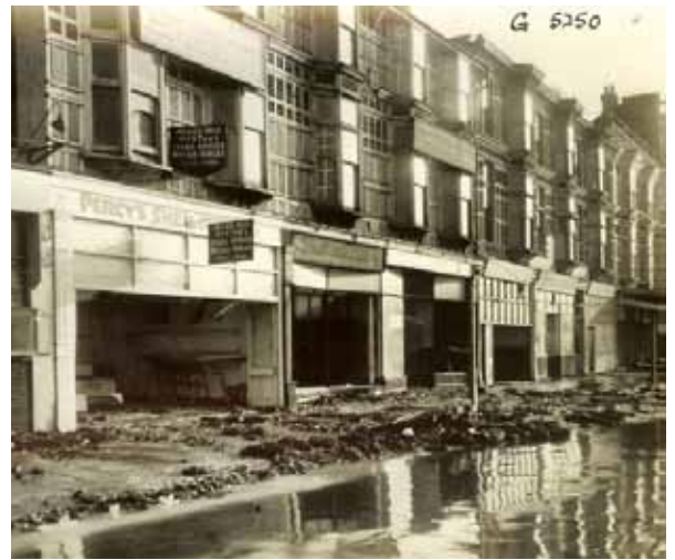
Flood damaged Marine Drive (1953) © Margate Civic Society
