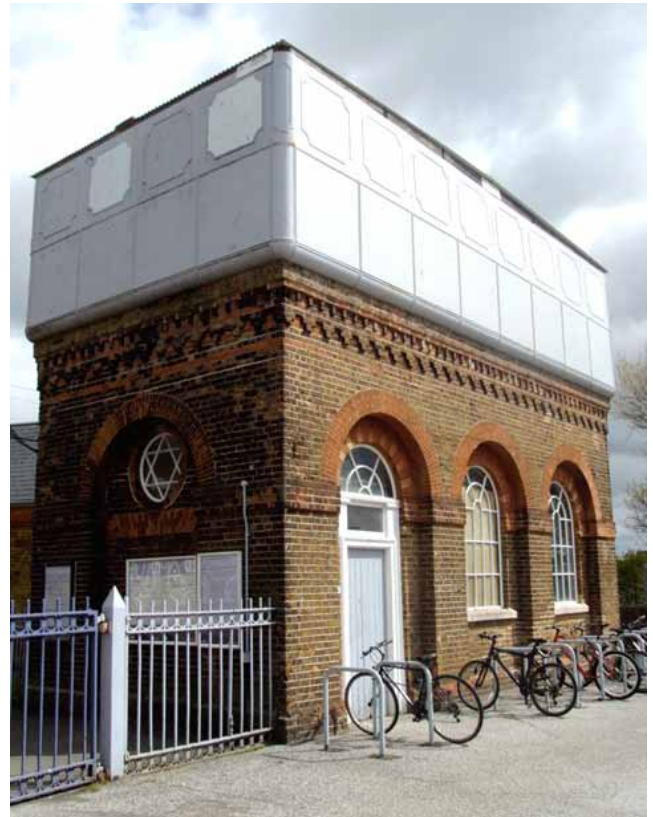
The classically-designed water tower Caroline Millar © RGS-IBG Discovering Britain
